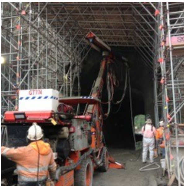
Geotech remote controlled head shotcrete machine, note long extension boom.
